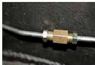
Proper Connection (Approved)
